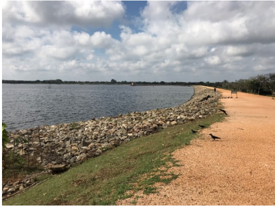
Fig 5: Riprap protection in the bund
