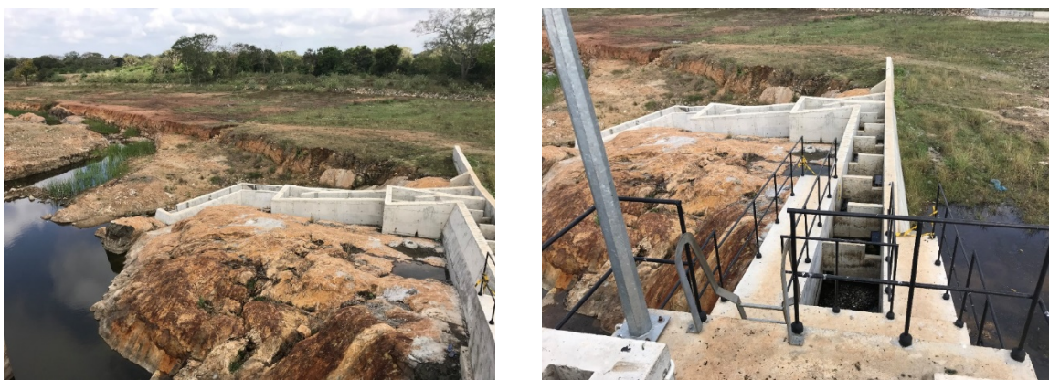
Fig. 10: Constructed fish ladder
