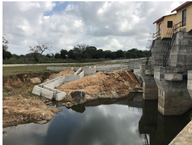
Fig 11: Construction of fish ladder closer to the spillway
