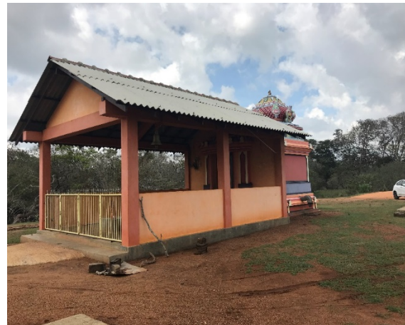
Fig 19: Newly Built Kovil
