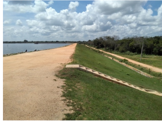
Fig 6: Turfing protection in the bund
