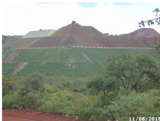
Figure 5 Process of coir matting in halfway on the dumps (overburden dumps)
