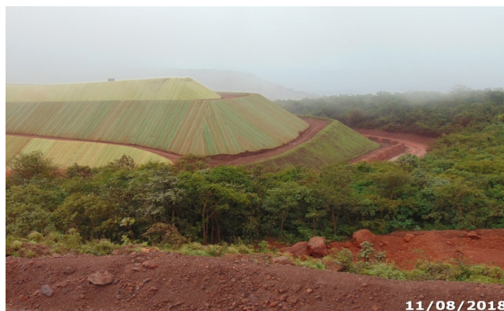
Figure 4 Coir mating/ geo-mating on waste dump
