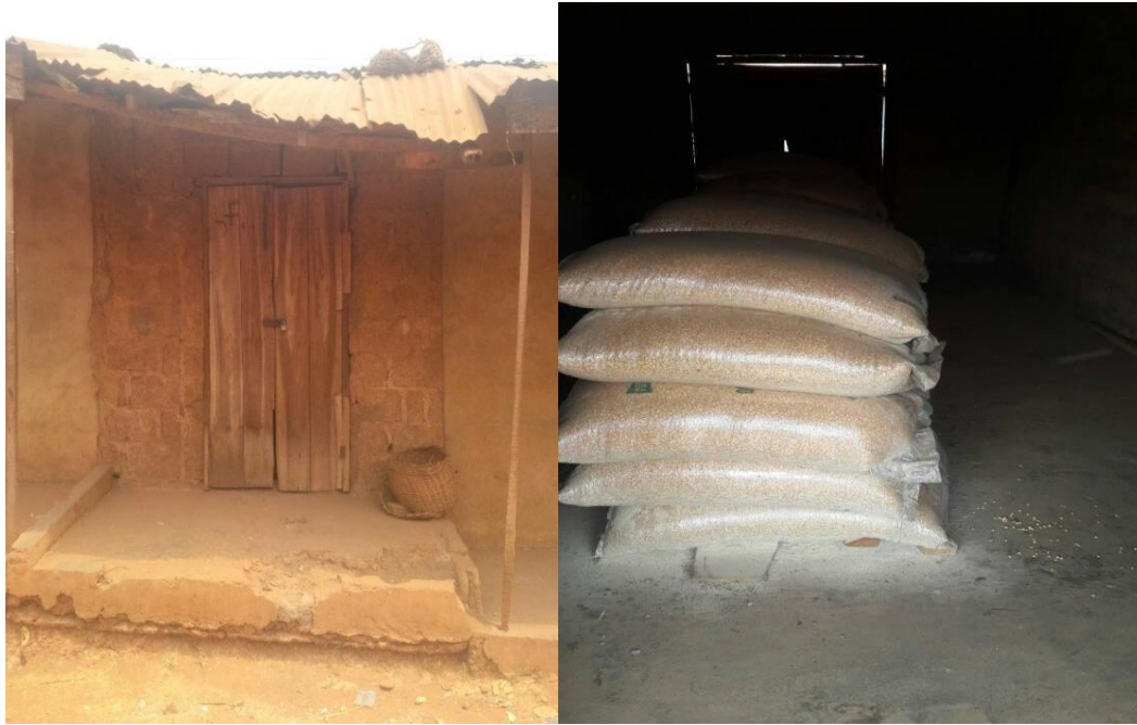
Figure 1: One of the Traditional Storage Practice (TSP) storehouses in the study
