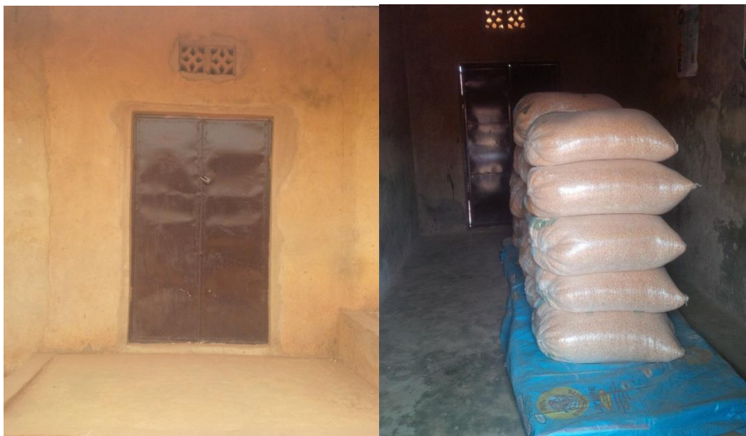
Figure 2: One of the Integrated Pest Management (IPM) storehouses in the study
