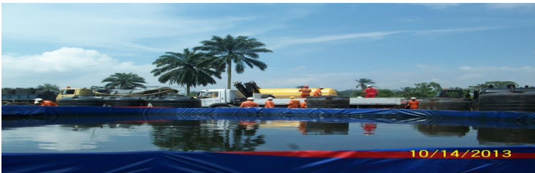
Figure 19: Temporary Storage Facilities for Recovered Spilled oil
