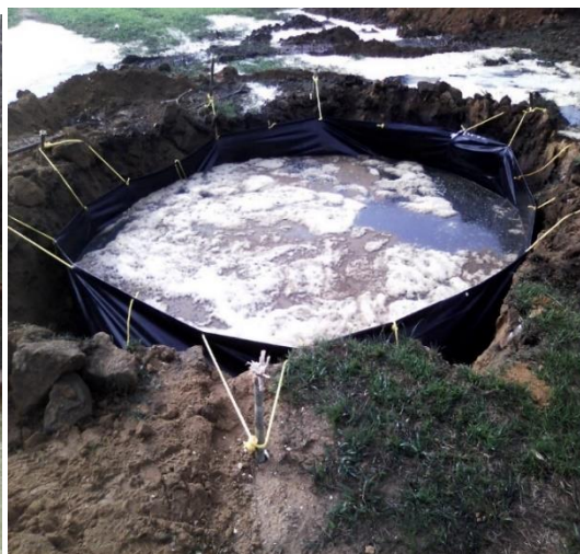
Figure 17: Contained Spilled Oil
