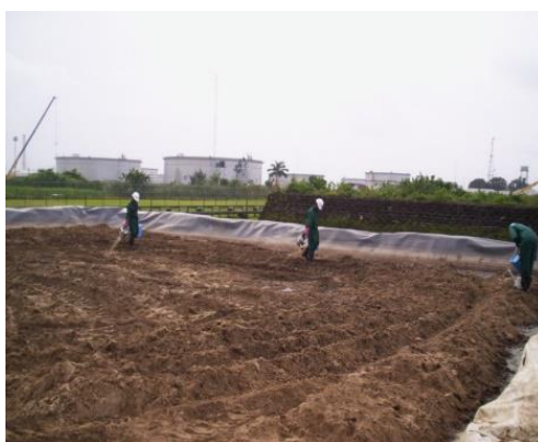
Figure 3: Broken Windrows and Nutrient Application
