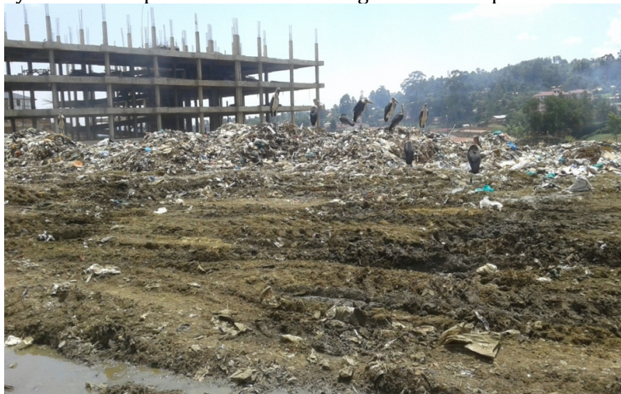
Plate 4.14: A section of Nyambara dumpsite under construction and scavenging birds
