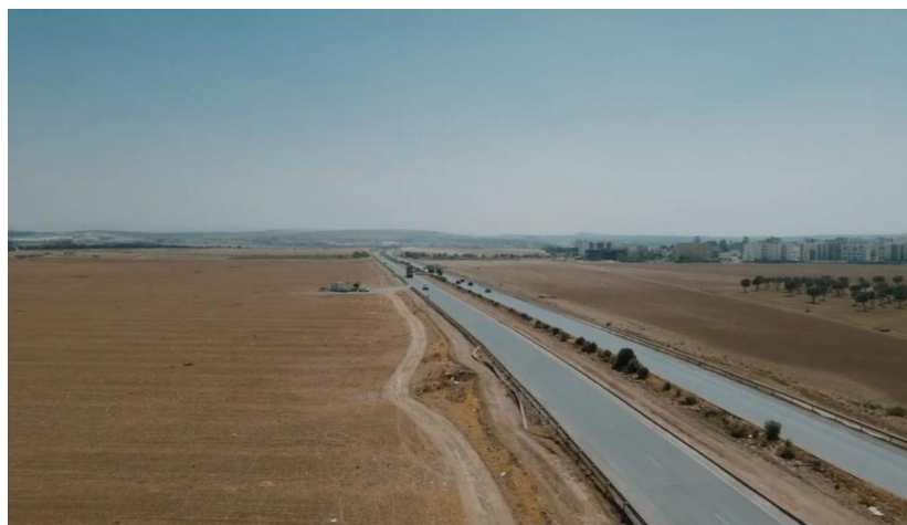
Figure 5: Photograph of the RE-MED pilot road on National Road No.3 in Tunisia, showing sections constructed with recycled materials alongside a control section using natural materials
