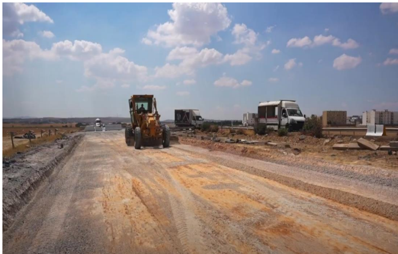
Figure 4: Photograph showing the preparation of the alignment for the RE- MED pilot road on National Road No. 3 in Tunisia
